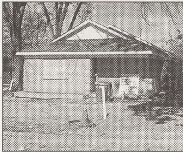
2122 Brown: new all brick, 3-bedroom, 2-bath- room house (just completed)
