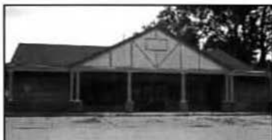
After: In September, renovations of the exterior are complete, except for landscaping
