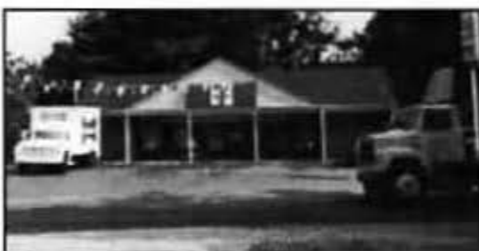
Before: Prior to VECA purchasing the building in 1996, it was operating as a 7-11 convenience store
