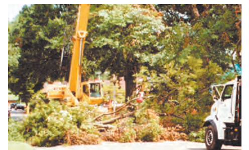
Cleaning crews following the Hurricane Elvis storm.
