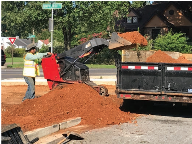
Memphis Landscape uses walking front loader to remove compacted substrate
