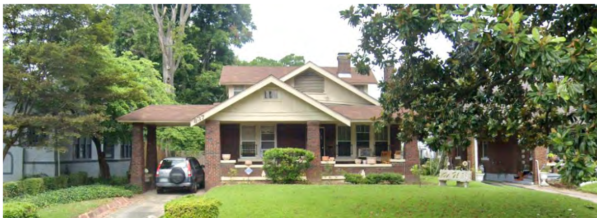
Image 3: (Above) Example of Craftsman Bungalow Style found in many structures throughout Vollintine Evergreen National Historic District Neighborhood Character Area
