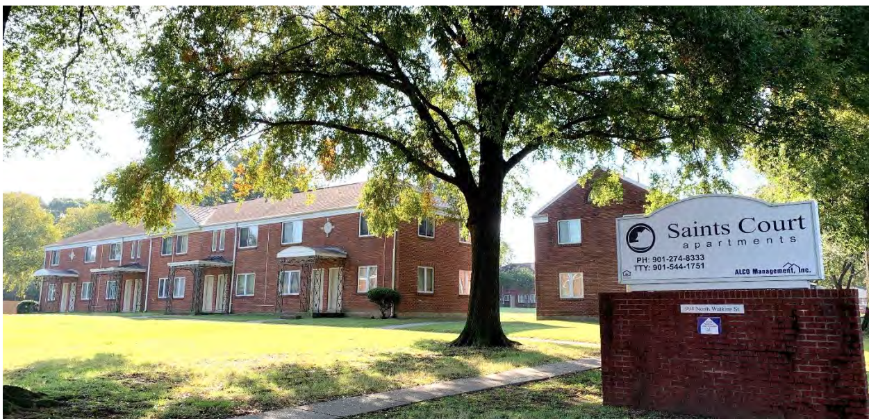
Image 40: (Above) The Saints Courts multi-family apartment complex consists of multi-story, attached buildings with very modest Colonial Revival detailing
