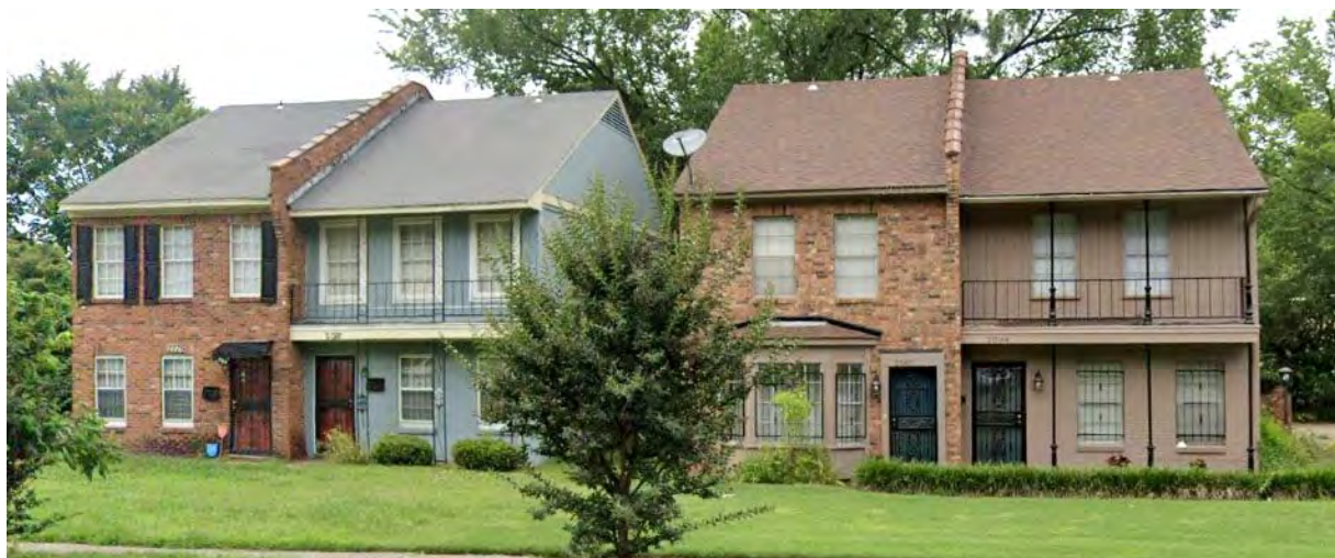
Image 60: (Above) One of two rows of ca. 1967 Contemporary style duplexes along Vollintine and University in the Cypress Neighborhood Character Area
