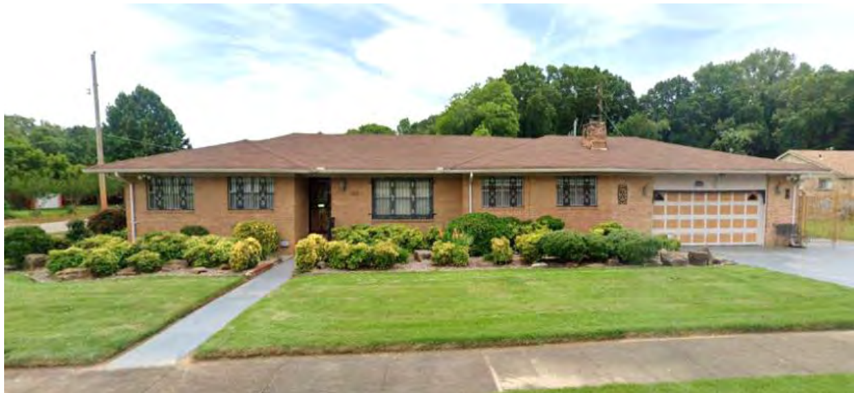
Image 50: (Above) Example of Ranch Style built in the 1970s in the Edward Avenue Neighborhood Character Area
