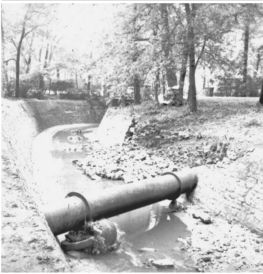
Figure 4: Lick Creek Channelization 1948 SOURCE: Board of Health Collection, Memphis-Shelby County Archives.
